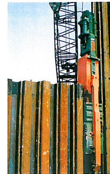
BELOW: HH7 with sound enclosure driving Larssen 6 in pairs, crane suspended mode, UK.
