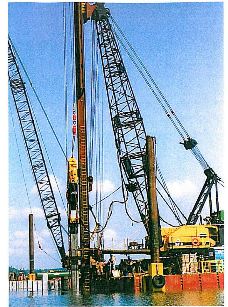
CENTRE: Crane suspended HH7 driving steel tubular piles 813 dia, UK.
